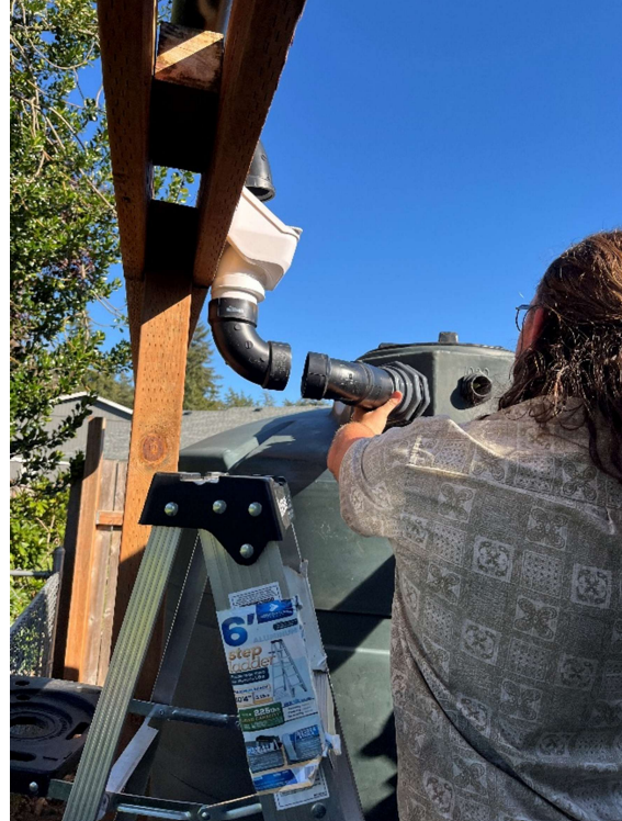
Dry fitting the plumbing
