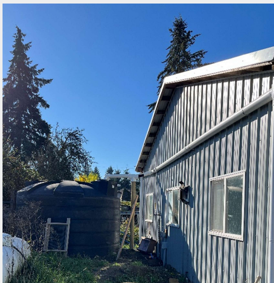
Completed rain tank collects from shop roof
