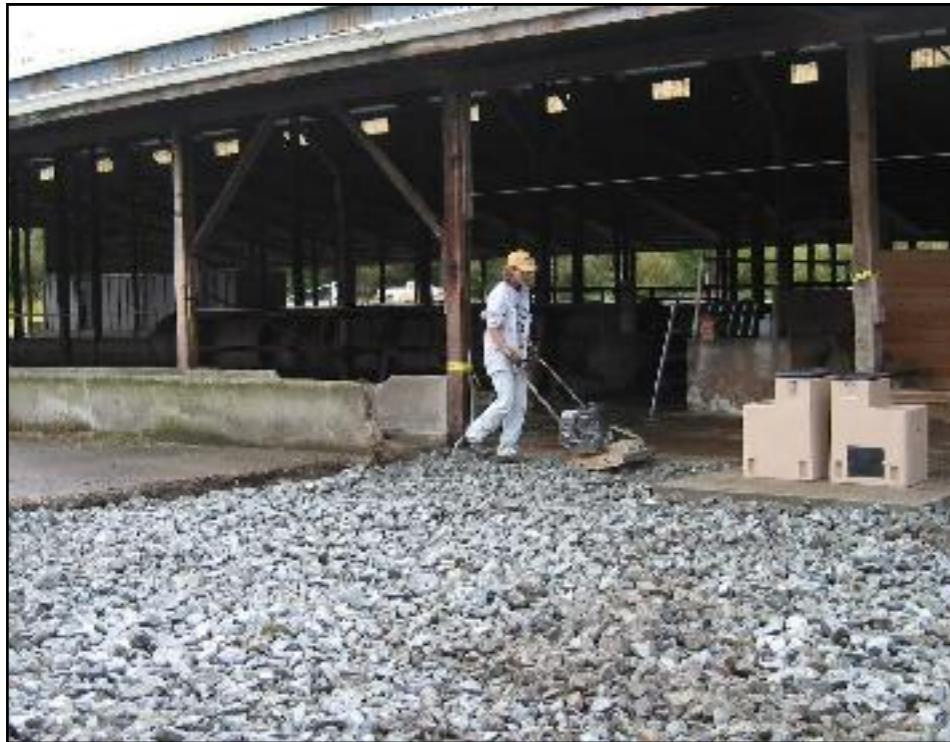
2. A FOUR INCH LAYER OF 2" - 4" CRUSHED ROCK (QUARRY SPALLS) IS SPREAD AND EVENED OUT WITH A COMPACTOR.
