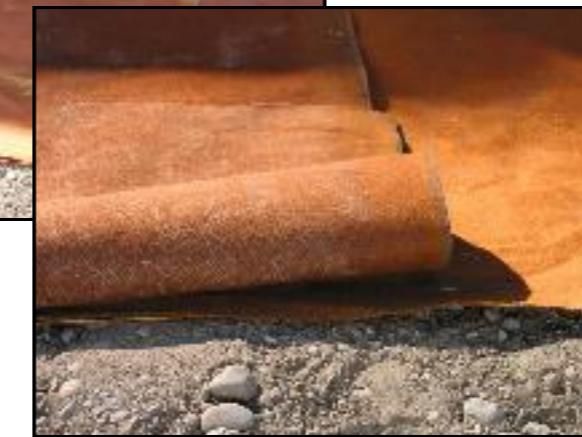
PROS: FABRIC HELPS TO DISTRIBUTE WEIGHT AND PREVENT THE MIXING OF SURFACE FOOTING MATERIAL WITH UNDERLYING SOILS ESPECIALLY USEFUL IN WET AND SANDY SOILS.
