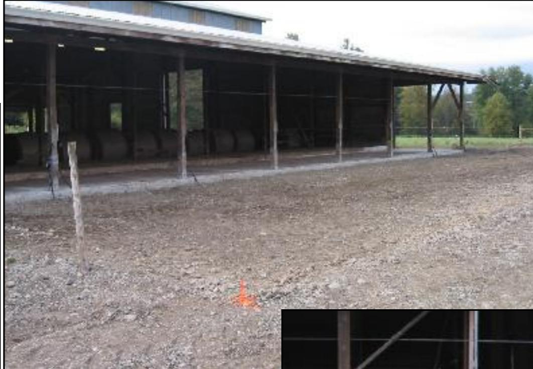
2. A FOUR INCH LAYER OF 2" - 4" CRUSHED ROCK (QUARRY SPALLS) IS SPREAD AND EVENED OUT WITH A COMPACTOR.
