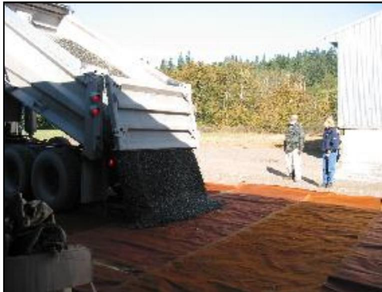
2. NON WOVEN GEO-TEXTILE FABRIC, CARPET OR PAPER BELTING IS ROLLED OUT. OVERLAP EDGES AT LEAST 12"-18". BORDERS OF THE FABRIC CAN BE KEYED IN, LOCKED IN BY RAILROAD TIES, OR EXTENDED BEYOND THE EDGES OF THE PADDOCK AND COVERED.
