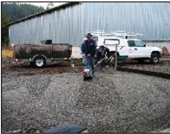
3. THE GRIDS ARE LAYED OUT AND SNAPPED INTO POSITION. THE GRIDS CAN BE CUT WITH A CIRCULAR SAW IF NEEDED. LEAVE A SMALL SPACE BETWEEN THE GRID AND WALLS.
