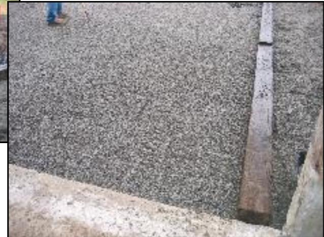
5. A FINAL 2" - 6" LAYER OF WASHED, COARSE SAND IS SPREAD OUT AND RAKED ON THE SURFACE.
