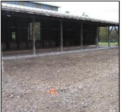
2. A 2" LAYER OF WASHED, CRUSHED 3/8" - 5/8" ROCK IS SPREAD, COMPACTED AND SMOOTHED.
